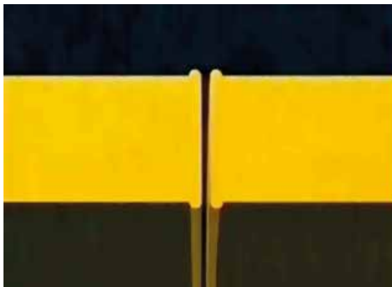
Figure 5: After the heating-up, closing the pipes face to face and joining them under pressure
