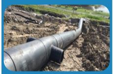
A typical landfill uses leachate collection systems to protect the water and the environment from landfill contaminants. These systems use a series of high-density polyethylene riser shafts, which must have additional pipe continuously added to the riser as the landfill soil cover increases in height. The characteristics of HDPE pipe and fittings allow these systems to be continuously modified as the landfill progresses.
